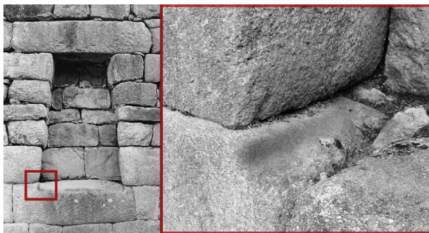
Fig. 9.14 The corner of a niche threshold in Sector 6B. Photo by A. Kubicka
