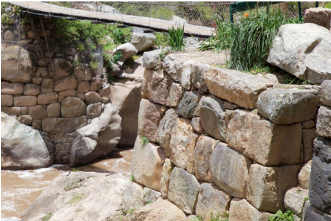
Fig. 11.30 Abutments of the Qoriwayrachina I bridge (Photo José M. Bastante)
