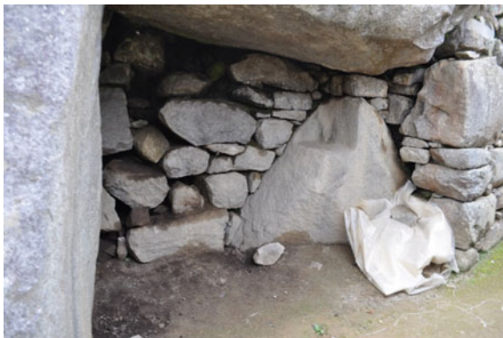
Fig. 7.28 The closed “cave” under the building placed in Sector Urbano
