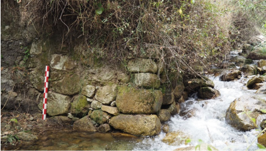
Fig. 10.9 Chachabamba stream channelling wall. Photograph by Dominika Sieczkowska
