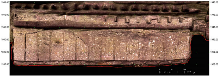
Fig. 9.10 El Fuerte de Samaipata. The back wall of a room in Sector S10—orthoimage from 3D laser scan. Elaborated by J. Kościuk
