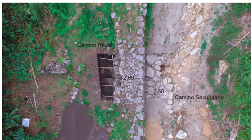
Fig. 11.14 Detail of the secondary road that is attached to and at a lower level than the main structure. The width is 2.50 (Photo Dennis Quispe)
