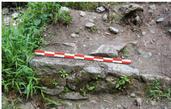
Fig. 11.23 Abutment of the Inka bridge in San Miguel (Photo José M. Bastante)
