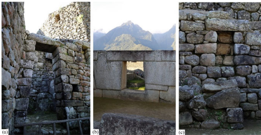
Fig. 4.12 a Doors, b windows and c niches at Machu Picchu. Photograph by the authors
