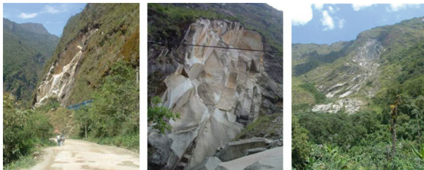
Fig. 2.13 One of the main rock falls in the area along the railway from Aguas Calientes to Puente Ruinas
