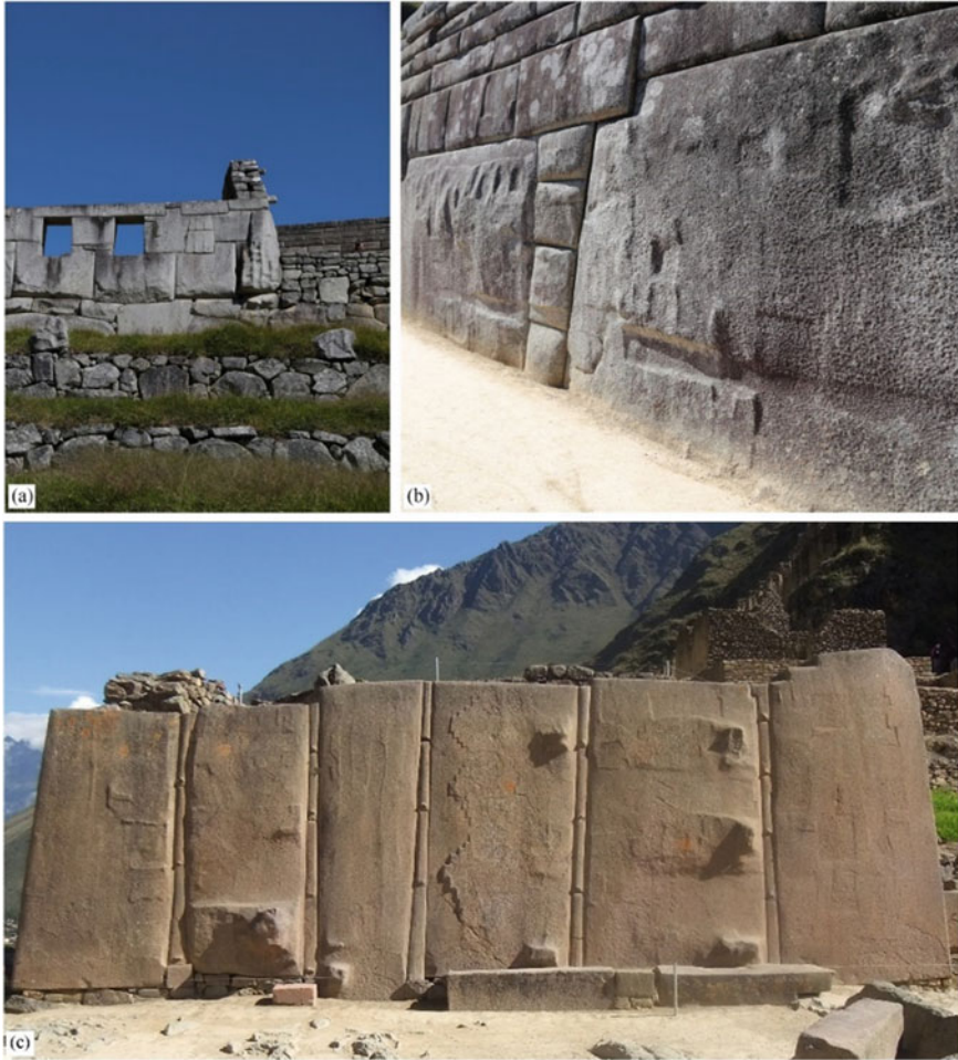
Fig. 4.7 Marks of extraction from larger blocks, visible at Machu Picchu in a the Temple of the three windows and b Main Temple and c in the Temple of the Sun in Ollantaytambo. Photos by the authors
