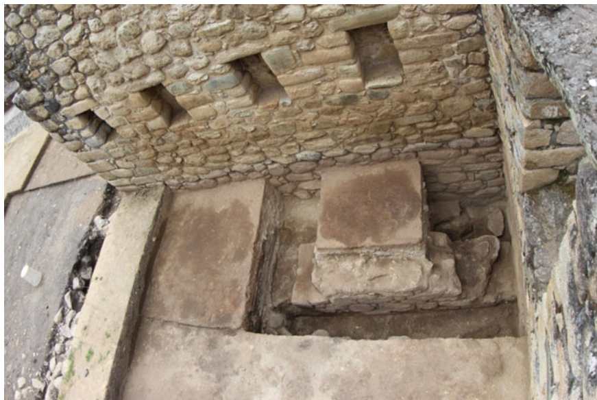
Fig. 10.12 Underground wall corresponding to the initial stage of construction of the monument. Photograph by Emerson Pereyra, PIAISHM archives
