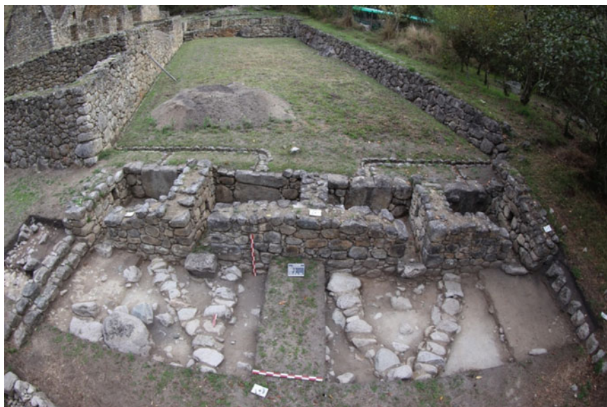
Fig. 10.8 Baths from the bottom of sector I (UE 01-2016). Photograph by Emerson Pereyra, PIAISHM archives
